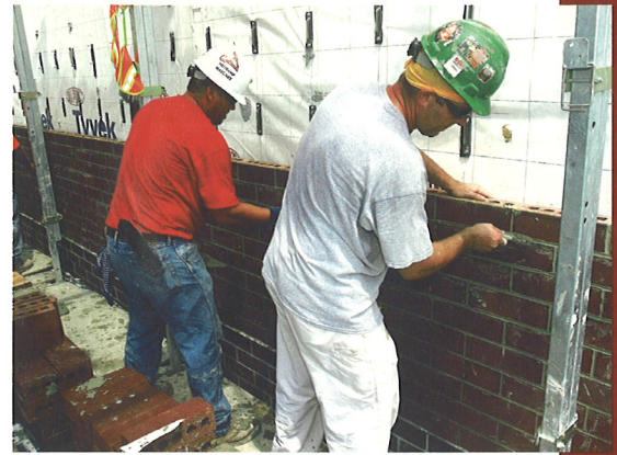
BRICKLAYERS FROM HEITKAMP MASONRY LAYING BELDEN BRICK OUTSIDE THE 22ND FLOOR.
