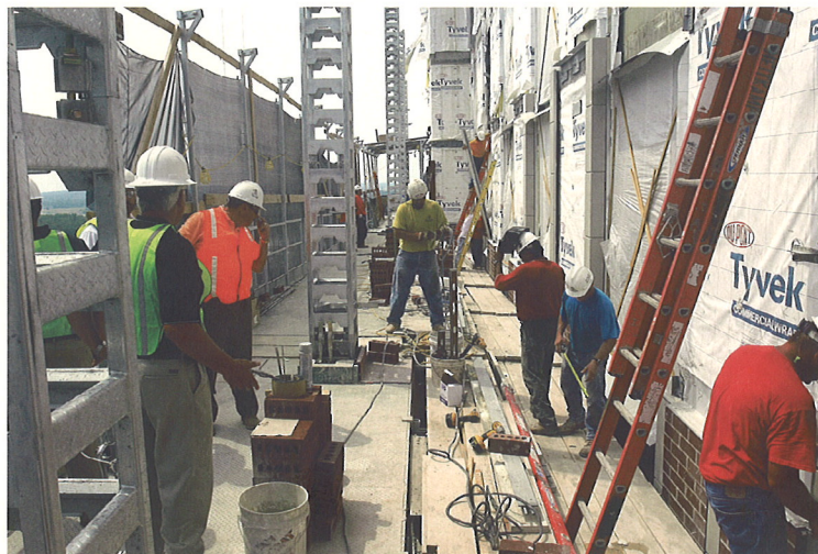
TWO HUNDRED FEET ABOVE THE MISSOURI RIVER, WORK ON THE HOTEL’S EXTERIOR PROCEEDS IN SMOOTH PRECISION.
