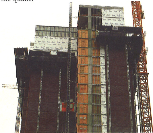
HYDRO MOBILE SCAFFOLDING PROVIDES A SAFE WORKING ENVIRONMENT WHILE HELPING TO SPEED THE PROJECT ALONG.
